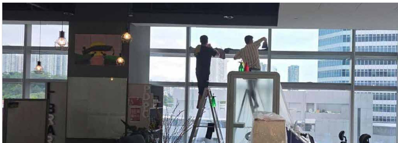
Solar Films Installation
