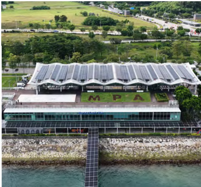
Solar Panels at Marina South Pier
