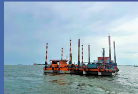
Soil investigation works for Tuas Port Phase 3 using jack-up barge
